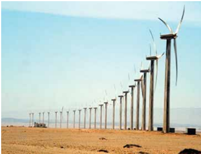
Zafarana Wind Farm, Egypt 8
